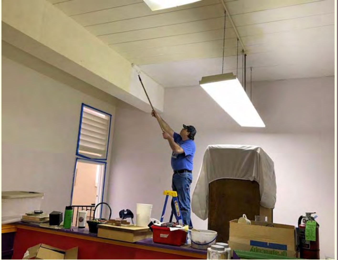
Classroom repainting continues -- Michael gets to do the high parts.
